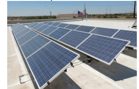
Solar rooftop PV system
