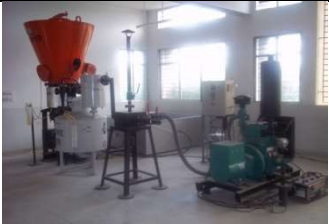
Biomass Gasifier Power system
